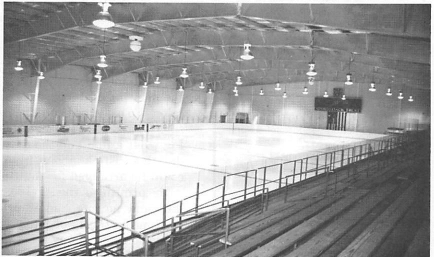
A clear span building enclosing a 100x200 ice surface.
